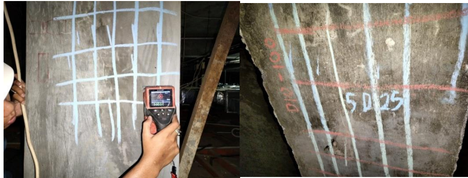
Figure 1. Existing column condition during field investigation
